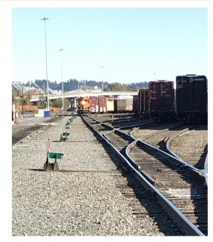
switches or derails that may be lined improperly. We must visually inspect the route in advance of these movements to ensure they are completed safely.
